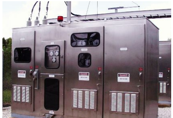
2.4 MVAR 15 KV AUTOMATIC UNIT IN SS 316 ENCLOSURE
