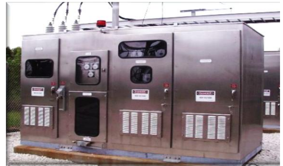
2.4 MVAR 15 KV AUTOMATIC 5 th HARMONIC FILTER IN A SS 316 ENCLOSURE
