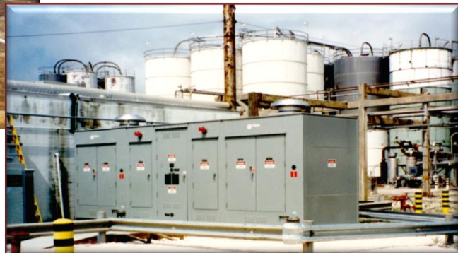
2.4 MVAR 15 KV AUTOMATIC 5 th HARMONIC FILTER IN A SS 316 ENCLOSURE
