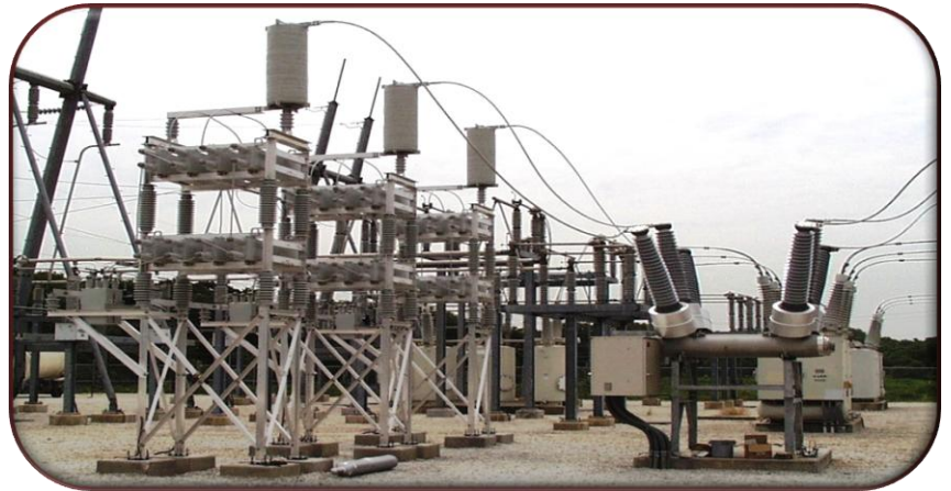
30 MVAR 138 kV, Substation Style Capacitor Bank.
