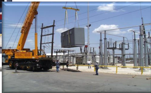
2.4 MVAR 7.2 KV 5 th Harmonic Filters for Induction Furnace Application
