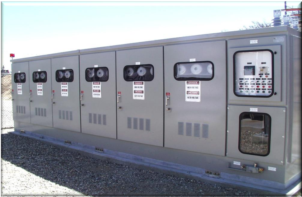
20 MVAR 12.47 KV, Six Stage Automatic Metal Enclosed Power Factor Correction Unit
